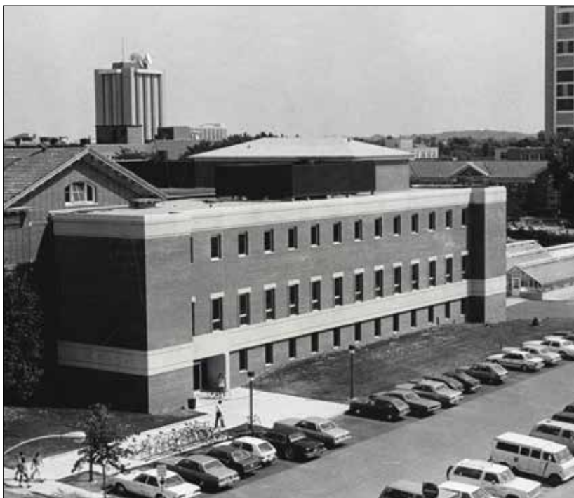
After remodeling and an addition, the Horticulture Building complex nearly doubled its laboratory and classroom area.
